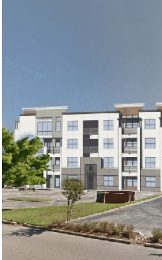
ALEXAN AT AUDUBON Location: Orlando, FL Developer: Cornerstone Number of Units: 357 Scope of Work: Kitchen, Vanities Status: In Progress
