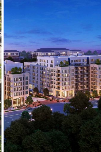
CAMDEN BUCKHEAD Location: Atlanta, GA Developer: Camden Number of Units: 365 Scope of Work: Kitchen, Bathrooms Status: Complete
