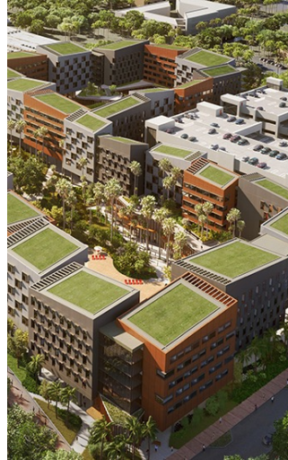
UNIVERSITY OF MIAMI STUDENT HOUSING Location: Coral Gables, FL Developer: University of Miami Number of Units: 442 Scope of Work: Kitchen, Vanities, Closets Status: In Progress
